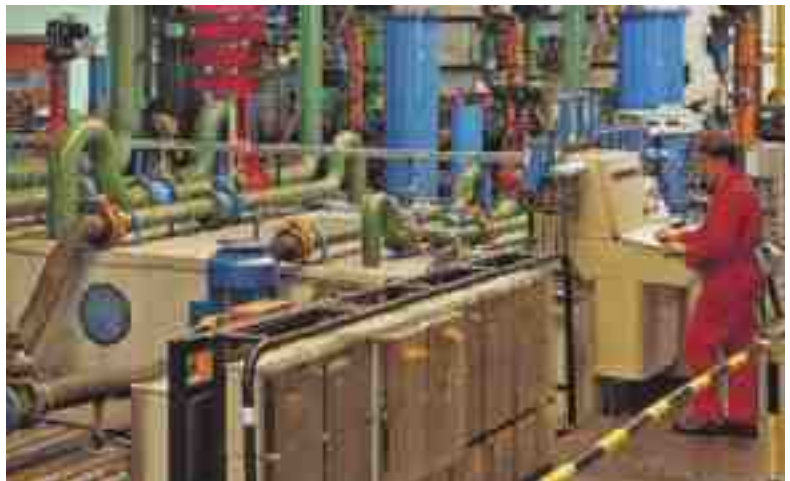
Test bed SPX Flow Technology in Assen, the Netherlands
